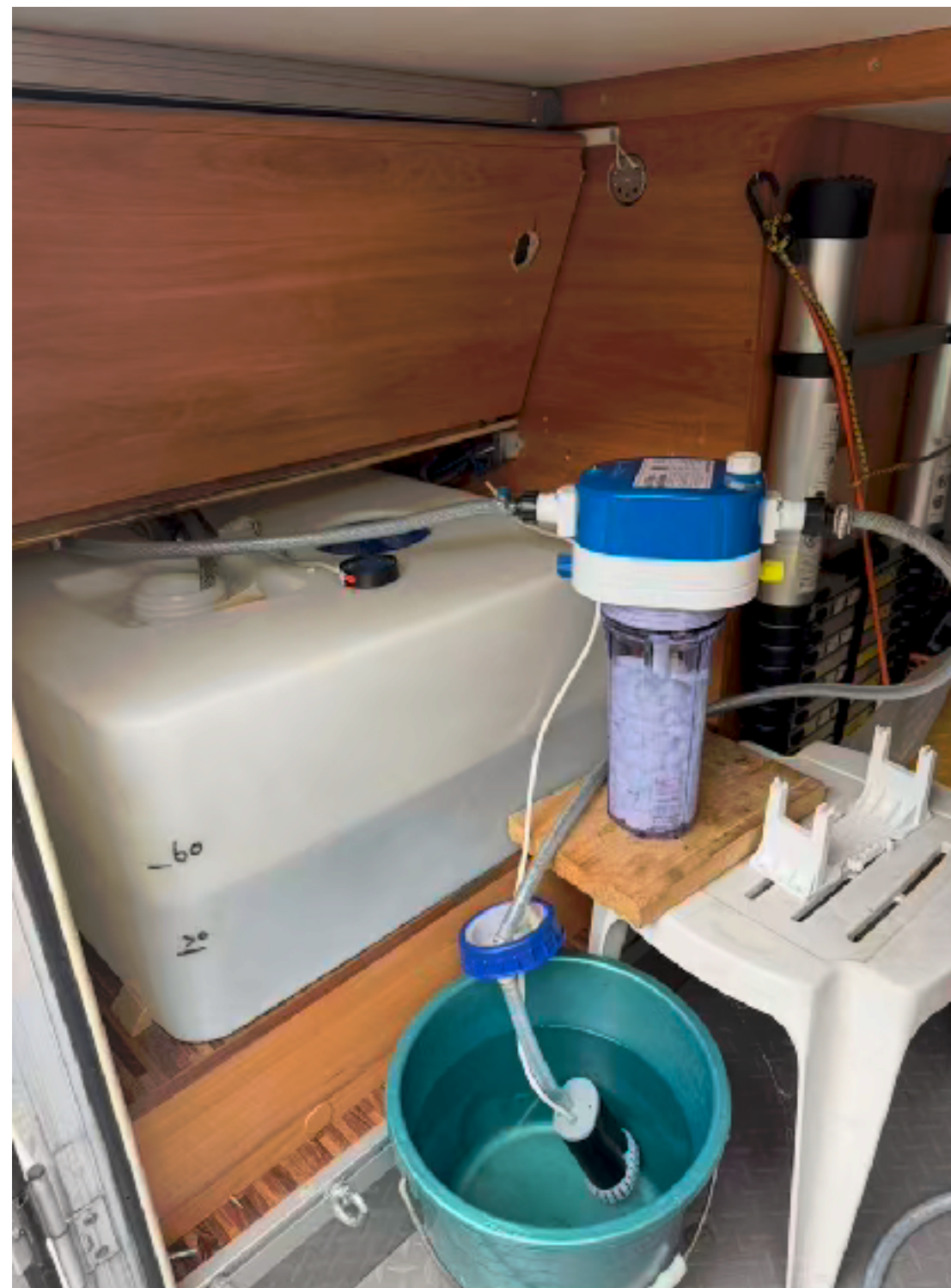
Disinfecting the old tank (which had not been cleaned for 8 years)
