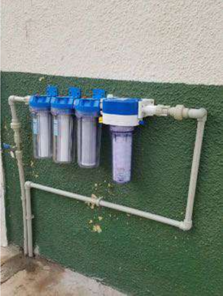
Installation, Sensiblu with 3 prefilters, rinsable 100 micron (protect Sensiblu from sand), replaceable 20 micron (reduce NTU) & 1 micron Cyst rated to prevent protozoa.
