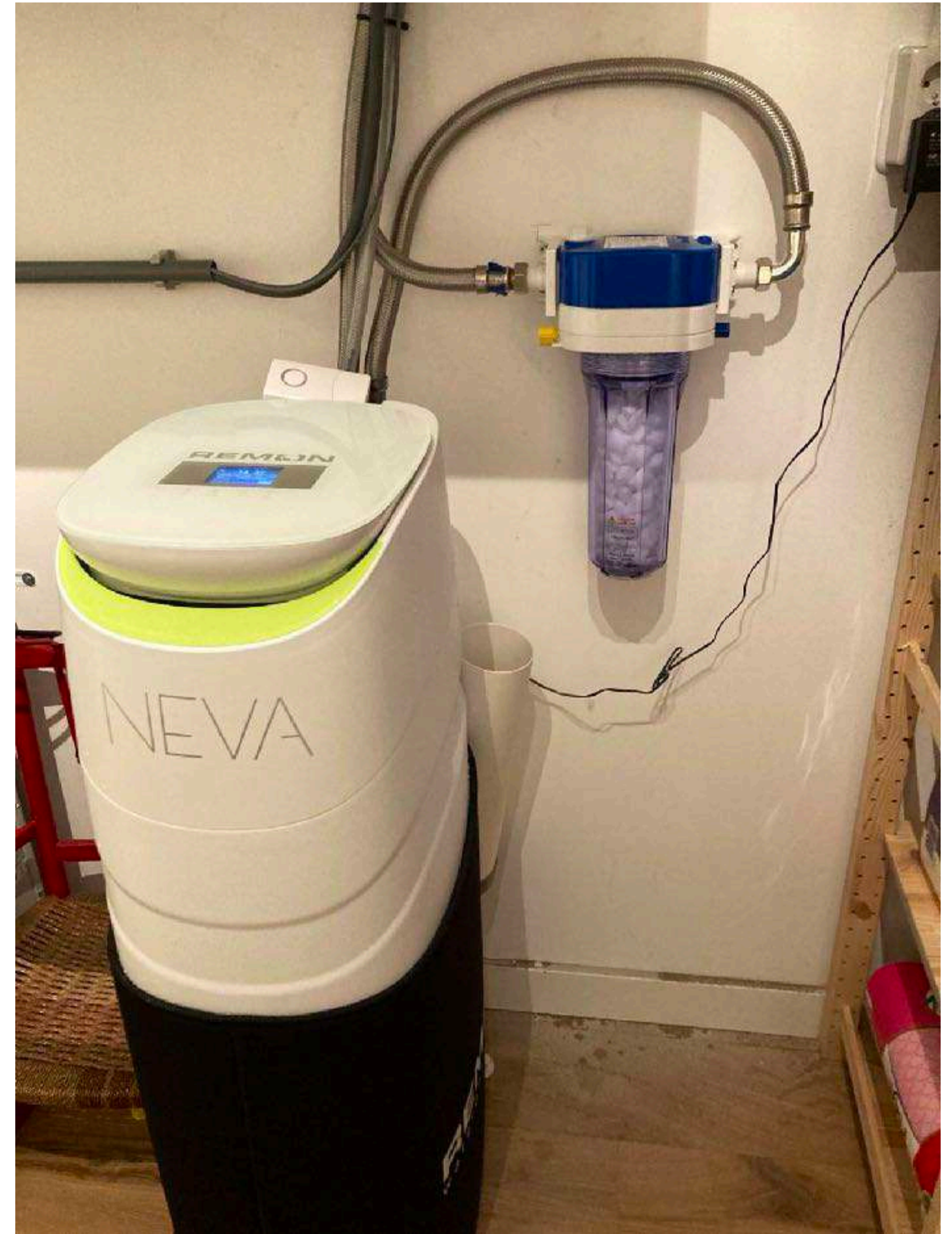
Whole house treatment, 1st Sensiblu, then through water softener device
