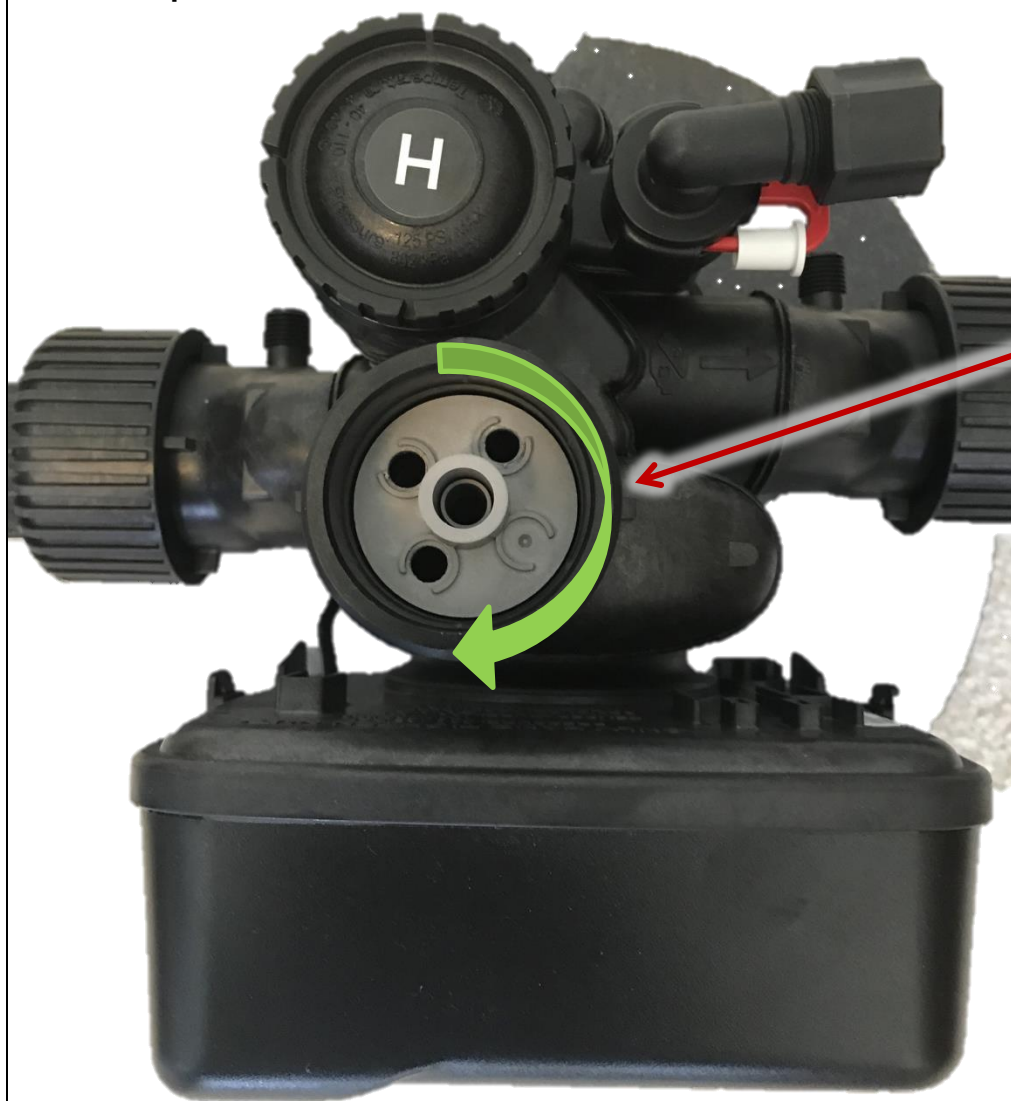
Top View of the WS1.5P Control Valve
